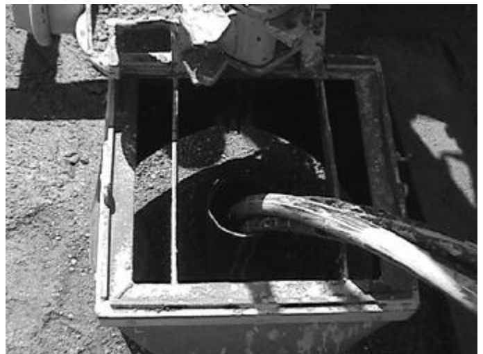
Inserting Plastic “U” tube in 4” Borehole
